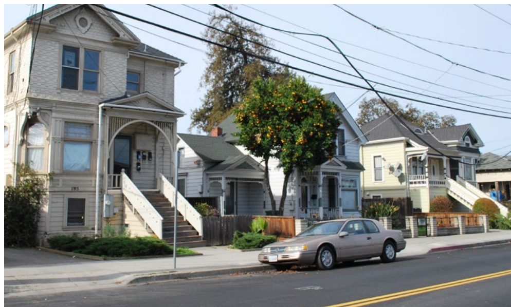
Because so much of downtown San Jose’s historic fabric is gone, what remains is an important asset. This block of Victorian homes on Autumn Street, just north of the Arena, should be preserved and incorporated into the redevelopment vision for the Diridon Station area.
