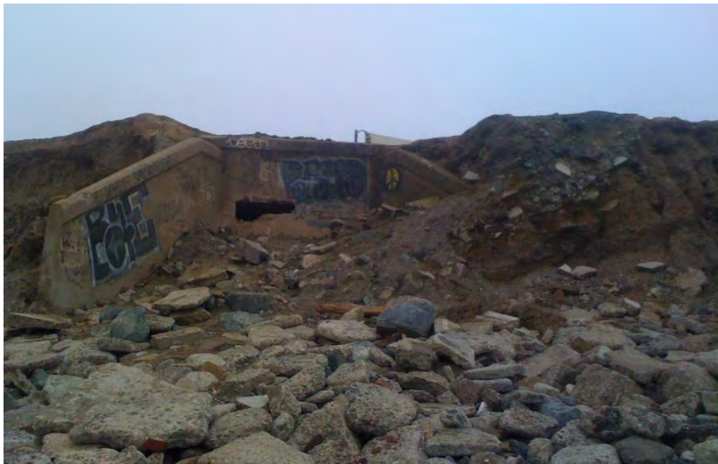
Figure 8: The inscription says “1926 200’ EXTENSION”. This structure, apparently constructed in the early 1900s has just recently emerged from the eroding fill at the south Ocean Beach “erosion hotspot.” A parking lot previously extended seaward on fill covering this structure. This headwall location corresponds to a location just north of the building in Figure 7, and about 200’ seaward, beyond the roadway and in the beach. Photo Battalio April 2012
