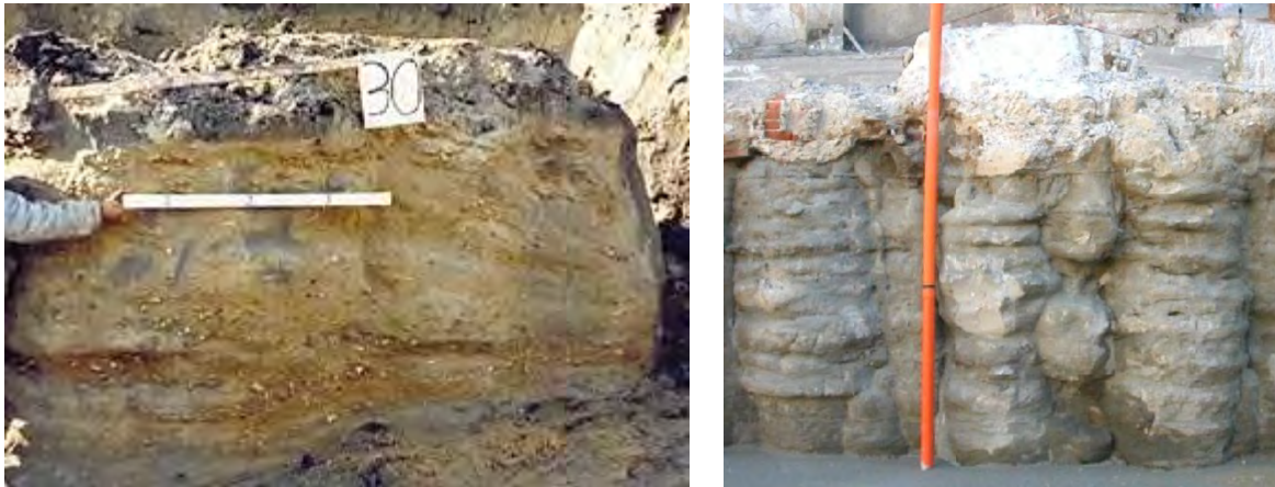
Figure 5 – Typical Soil-Cement Wall Examples – Jet Grout shown
