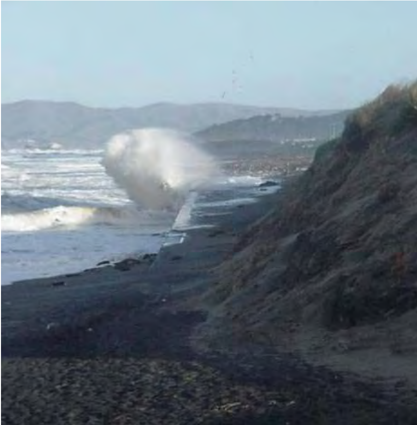
South end of the Taraval Seawall, near the end of Santiago Street, circa late 1990s, eroded conditions eroded conditions following the 1997-98 el nino winter. Photograph: Bob Battalio.
