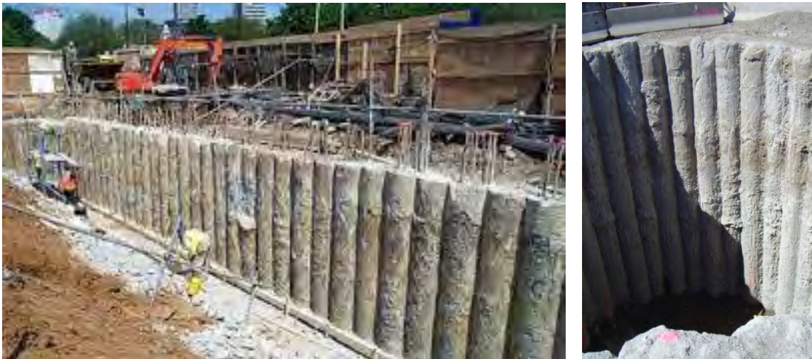
Figure 1 – Typical Pile Wall Examples
