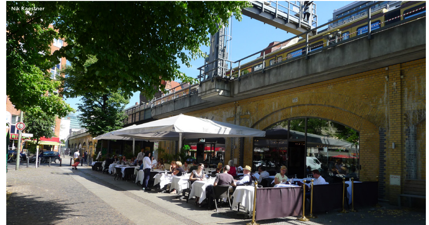
In Berlin, rail grade separations are integrated with neighborhoods.
